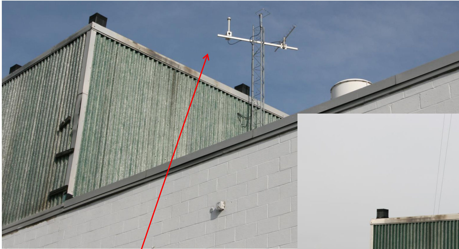
GPS antenna, 2 meter Omni antenna and 902 Yagi pointed at Phila.
